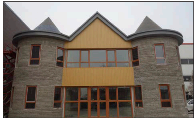
Fig. 11: 3D printed villa in China (Hossain et al., 2020)
