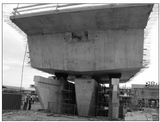
Fig. 8: Completed starting segment with anchor heads of transversal prestressing supported by stabilizing concrete walls
