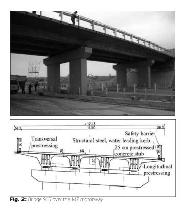
experimental purposes over the M7 motorway in 2006 (*Fig.* 2). The superstructure lies along a curved horizontal layout in varying (2.43-0.72%) longitudinal slope and constant 6% superelevation with 11.0+17.5+18.5+13.0 m spans. The 250 mm thick deck slab was monolithically built on a system of transversal and longitudinal beams (gridwork). The longitudinal beams as well as the deck slab in the transverse direction were internally post-tensioned by unbonded tendons.
