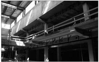
Fig. 4: Corridors of the mall lying on precast cantilevers
