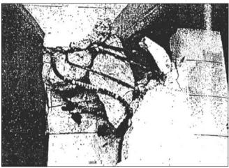
Fig. 21: Example of shear failure in an unexposed concrete column due to the thermal expansion of the fire exposed floor connected to it (fib, 2007)
