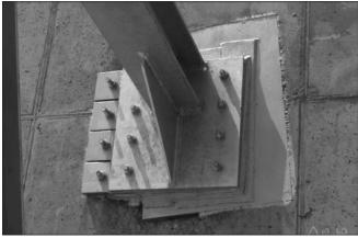
Fig. 12: Penthouse cantilever corrected joint
