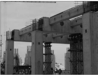
Fig. 10: Precast structure of the slab before concreting with temporary shoring structures
