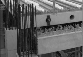
Fig. 10: Dead load reducing light fills between the ribs of the panels
