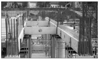
Fig. 3: Column-beam-slab joint in the mall
