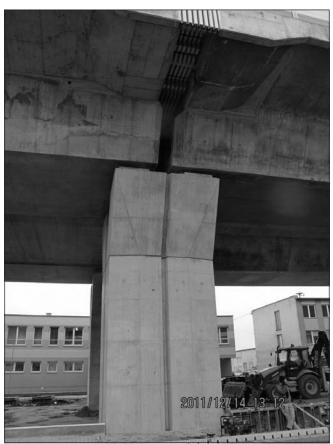
Fig. 5: Common pier 21 with expansion joint
