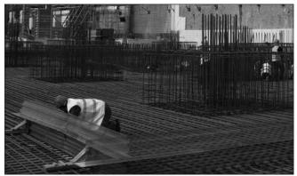
Fig. 2: Construction joint in the raft
