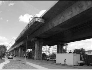
Fig. 14: Final works on DC1 bridge part: making of the curbs
