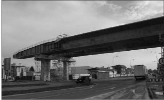
Fig. 7: Pushing of the DC1 bridge section above Nové Zamky road
