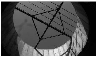
Fig. 11: Rotunda compiled with precast wall elements
