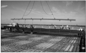
Fig. 11: Placing BAMTEC reinforcement on precast formwork elements
