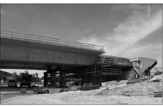
Fig. 10: Construction of the last segment of DC2 at abutment 26 in hanged formwork
