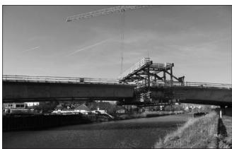
Fig. 11: Connection of the two arms of the DC2 bridge section above the river
