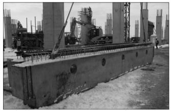
Fig. 9: 100 cm deep secondary girders with upper reinforcement before assembling on site
