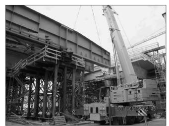
Fig. 13: Disassembly in pieces of the launching nose of DC1 just before reaching the common pier
