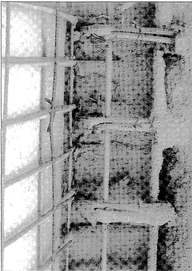
**Fig. 6** Anchorage of the welded wire mesh
