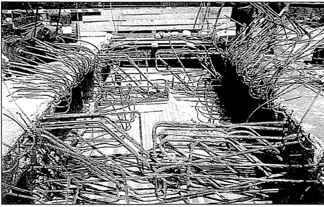
**Fig. 2** Dismantled Gerber hinge
