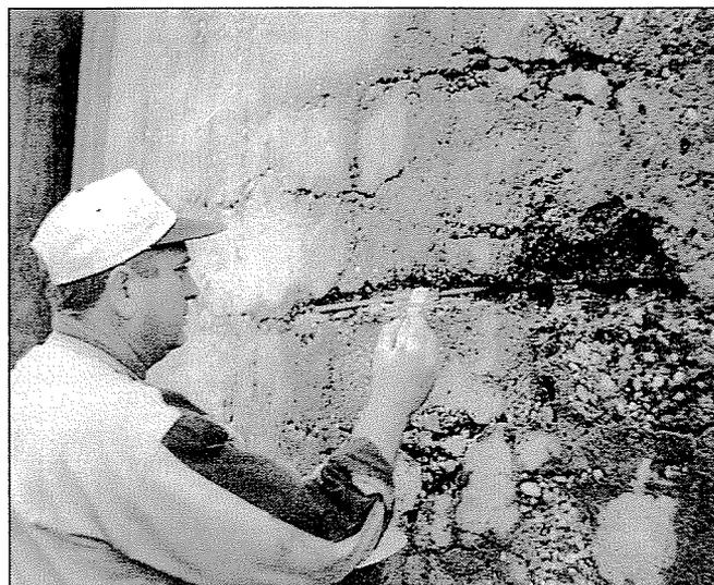
**Photo 1** The wall of the silo after sand blasting and the corrosion protection of reinforcing bars
