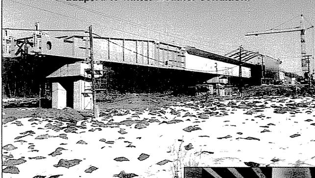
introduction. A number of up-to-date, monolithic bridges with spare hollows were constructed on the section by-passing the city of Győr of the motorway M1. An important result of the technologic development was the introduction of the so-called incremental launching method. In the period from 1989 up to now yet 22 bridges were constructed by this method, mainly on the base of the own designs
